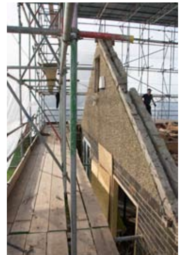
PICTURES: A watertight membrane was erected around scaffolding while the first floor was added. To make it easier to plan individual rooms, Clare, a graphic designer, marked photographs of the work in progress.
